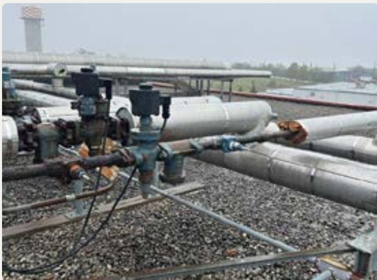
➤ The failed valve was replaced by a new one
