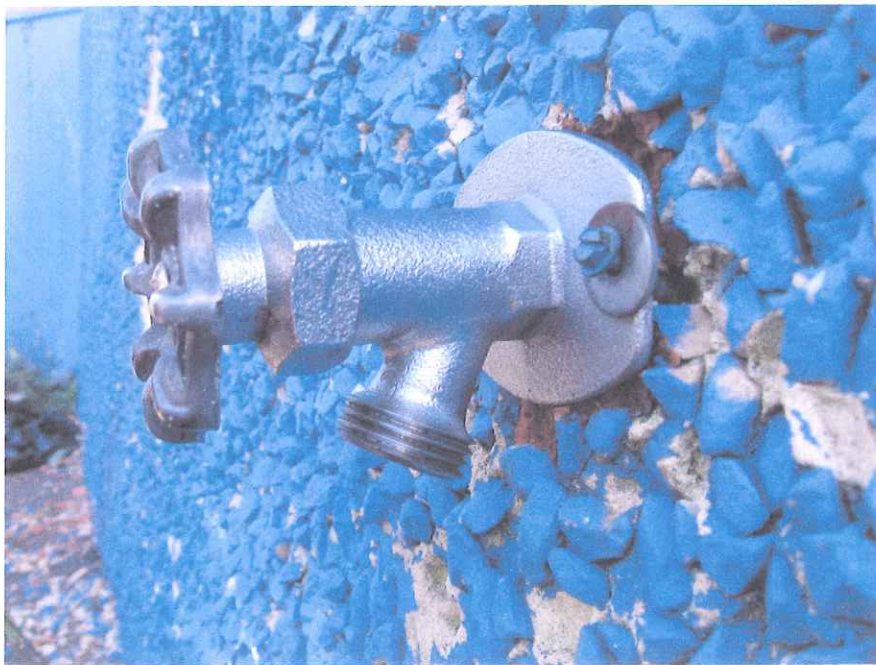
Extra Fire Protection: Fire Extinguisher located next to Propane Dispenser. Water Source by garage door West side of building (can be used to cool tank etc.)
