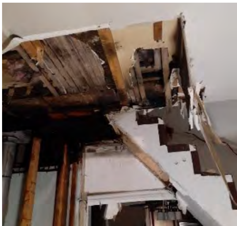
Figure 22: Staircase to second floor
