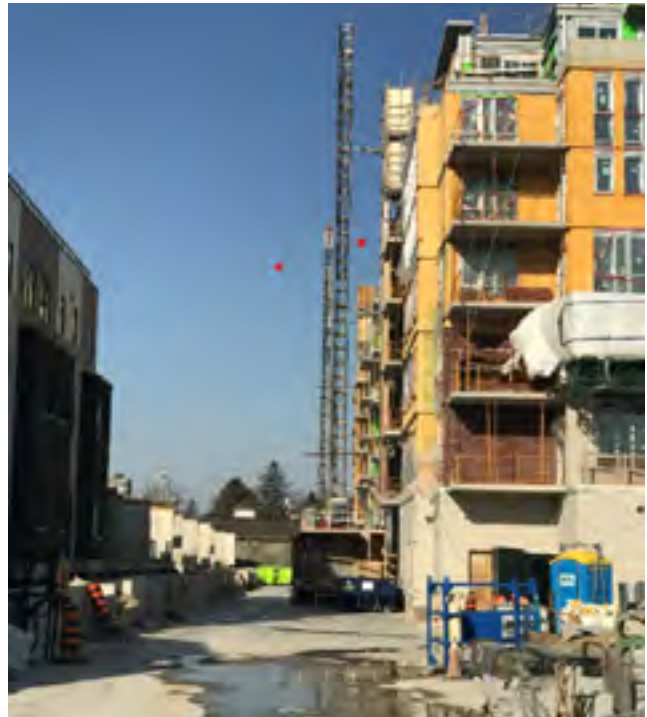
Figure 15: View of construction hoist
